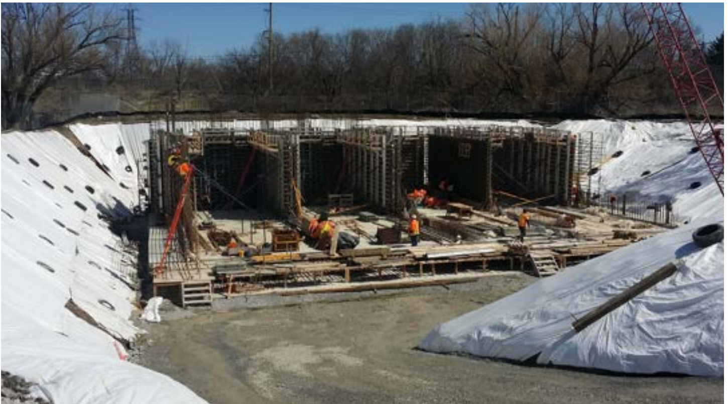
Figure 5: Glengarry Road CSO Tank
