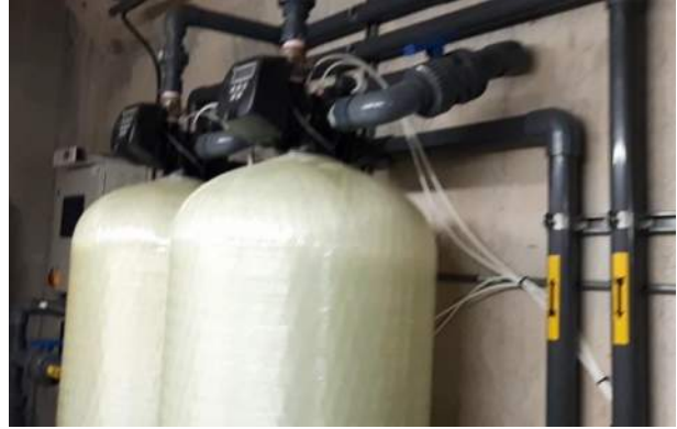
Figure 10 – Splash Pad Water Softeners
