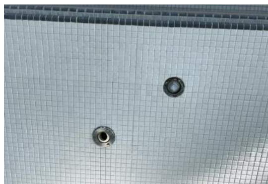
Figure 31 – Main Pool Return and Vacuum Fitting
