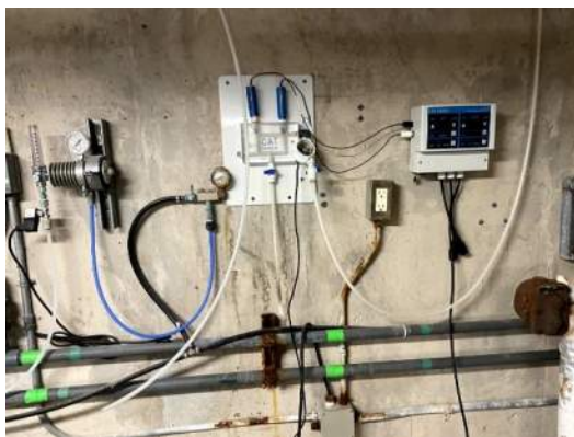
Figure 11 –Chemical Controllers
