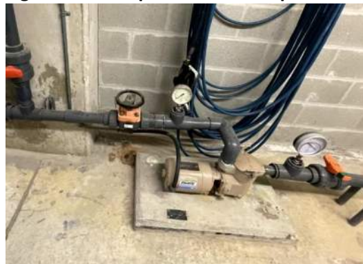
Figure 6 – Vacuum Pump
