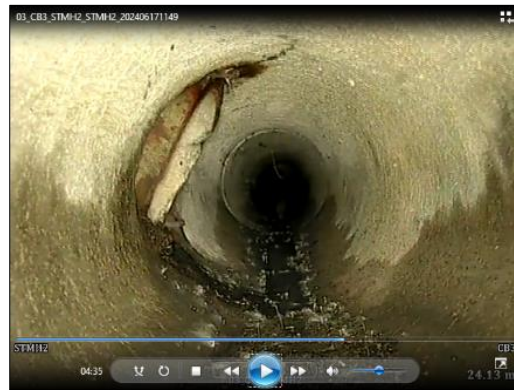
Photo C40: Lead CB 3 to STMH 2: Connection from CB 4.
