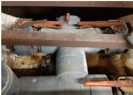
Figure 15 – Corroded Valves
