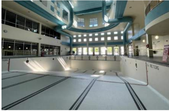
Figure 22 – Main Pool Tank
