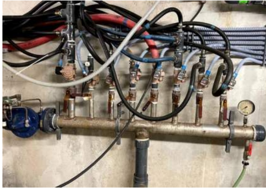
Figure 13 – Splash Pad Feature Return Piping
