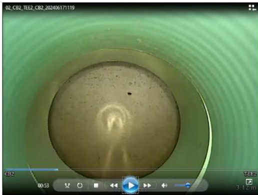
Photo C39: CB 2 Lead: Connection to storm trunk sewer.
