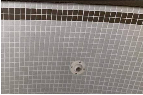
Figure 32 – Typical Whirlpool Return Fitting
