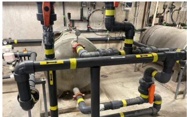
Figure 8 – Whirlpools' Horizontal Sand Filters
