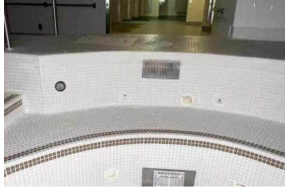
Figure 33 – Typical Whirlpool Vacuum, Equalizer, Hydrojet Fittings
