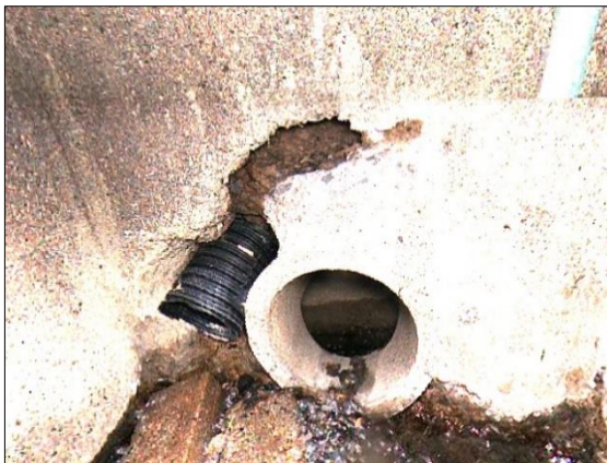
Photo C50: CB 4: Weeper Connection
