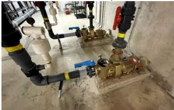
Figure 5 – Whirlpools’ Hydrojet Pumps
