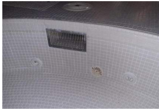
Figure 29 –Typical Whirlpool Skimmers
