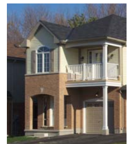
Putting a habitable storey atop the garage
