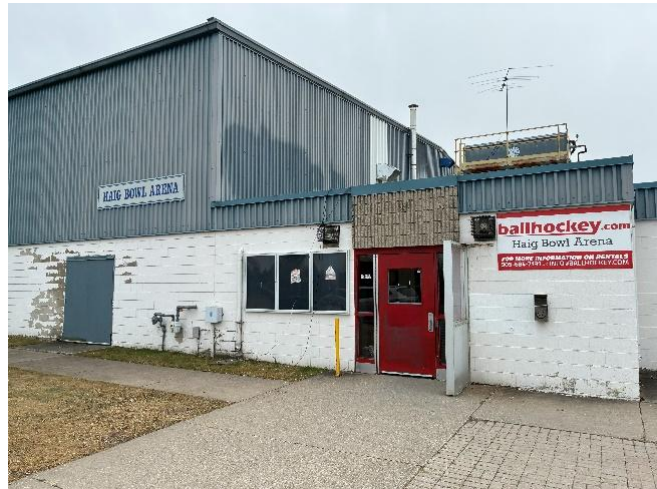
Photo 6. View of Haig Bowl Arena, looking south from Pleasant Avenue
