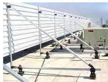
rooftop mechanical screening
