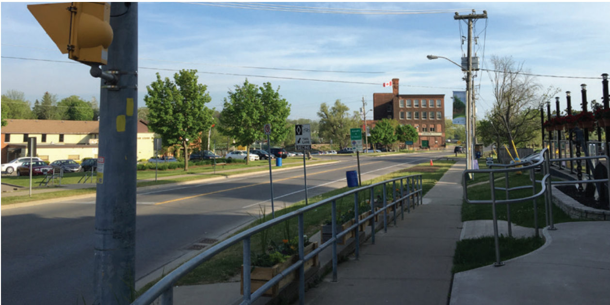
The alignment of Lakeport Road is recent and crosses over portions of the former Second Welland Canal, which passed west of the Maple Leaf Rubber Factory. Its current character allows open views to the water (Catherine Nasmith)
