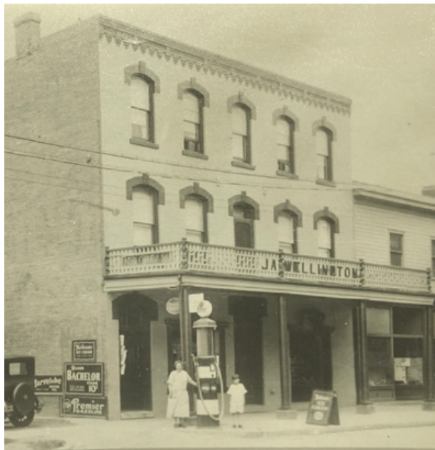
Lock Street c. 1920, Wellington Hotel: verandah, and sidewalk directly in front of hotel, but basic footpath to the east
