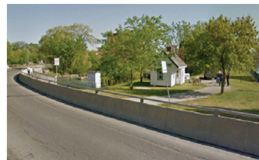
1c To the north to the Locktender's Shanty and the entrance to the Harbour Walk (Google Earth)
