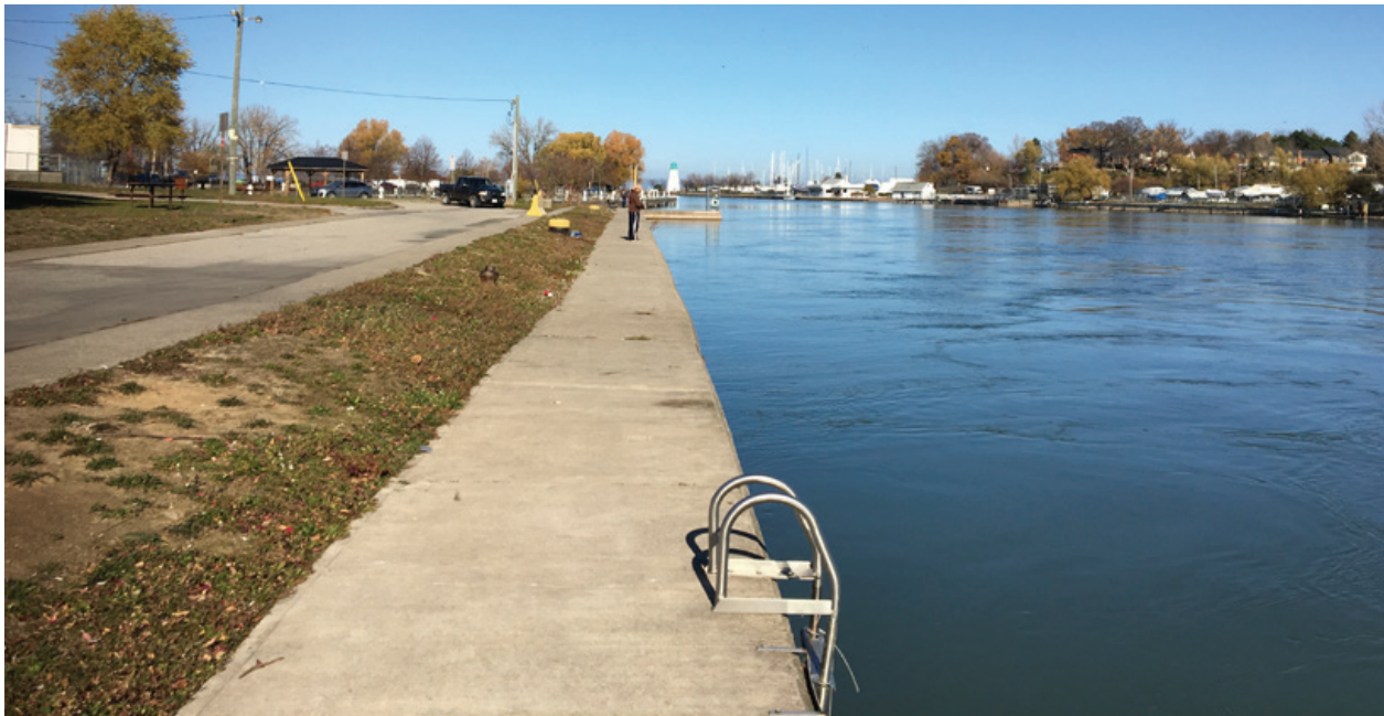
Utilitarian character of Third Canal edge, with marine equipment retained (Catherine Nasmith)
