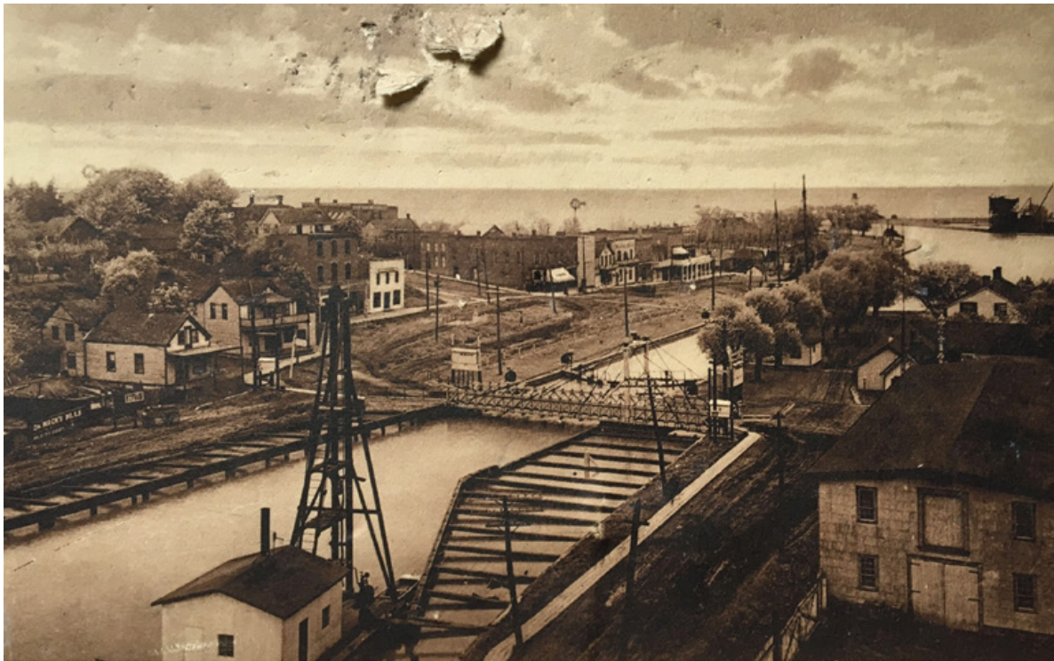
Historic Image of Second Canal showing random placement of buildings in relation to canal operations, and utilitarian character of the industrial areas, image courtesy of St. Catharines Public Library
