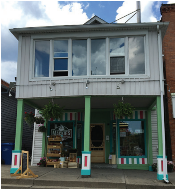
Two storey vernacular frame commercial building, 28 Lakeport Road, simple form with historic shopfront and veranda
