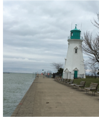
4g Inner Light House with Outer Lighthouse in background (Catherine Nasmith)
