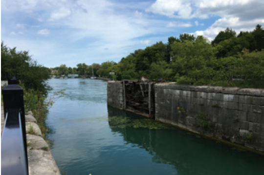
2d First Lock of Third Welland Canal (Catherine Nasmith)
