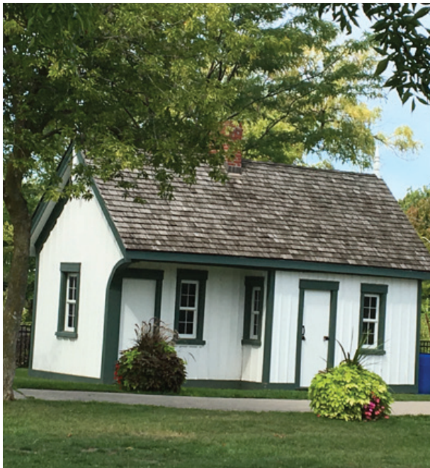
Wood shingles on the Lock keeper's Shanty (Catherine Nasmith)
