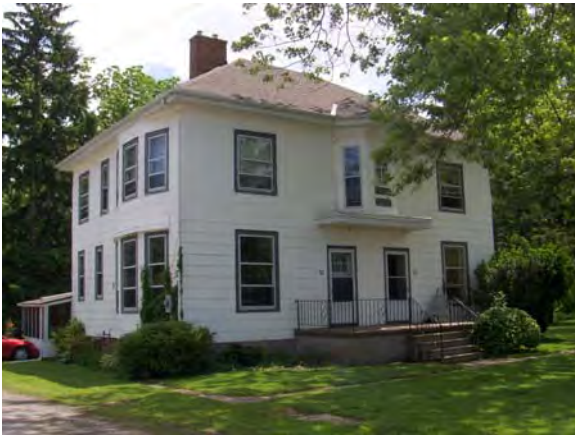
Figure 21: 21 and 23 Power Power Glen Road
