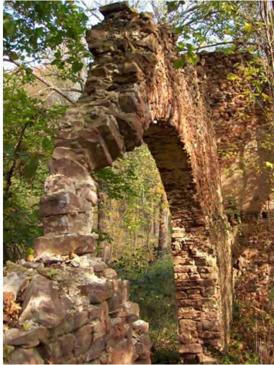
Figure 3: Remains of the arch marking where the gristmill wheel stood
