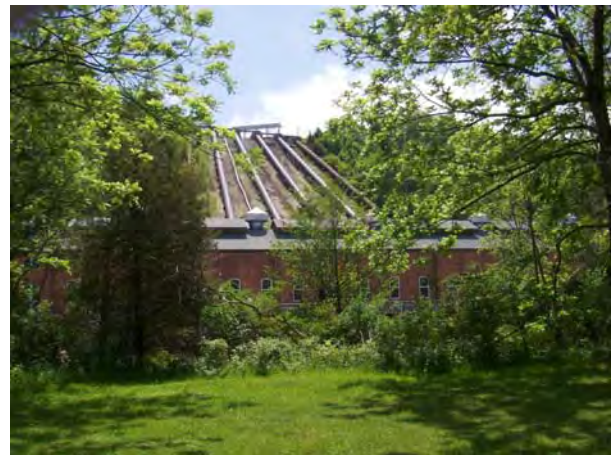
Figure 7: Decew Generating Station
