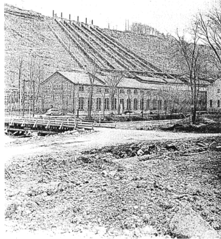
Figure 5a: Decew Falls Power Generating Station in 1940 2
