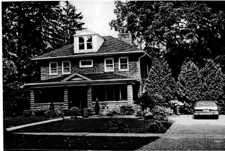
Upper: Stone is not used widely in Port Dalhousie buildings aside from foundation material. Lower: This example (100 Main Street) is the sole use of concrete block in Port Dalhousie.
